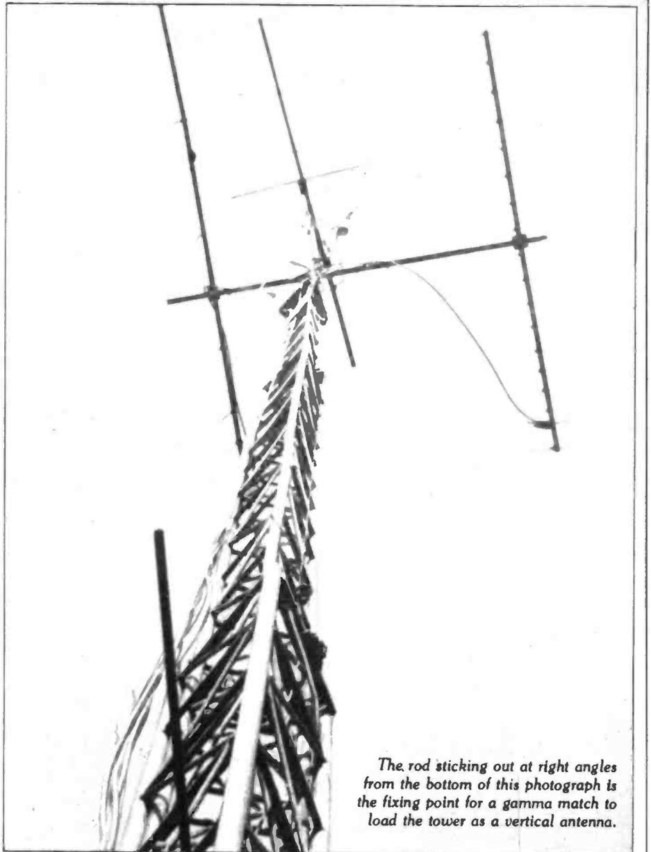
*The rod sticking out at right angles from the bottom of this photograph is the fixing point for a gamma match to load the tower as a vertical antenna.*
