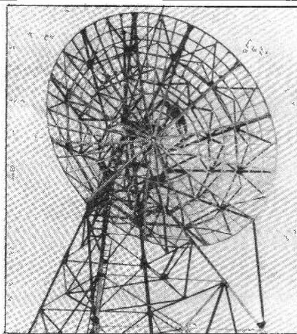
Construction work on the troposcatter dish at Mount Misery, Barbados. Similar aerials of 30ft diameter were used on the Start Point - Galleywood link. Photo: Marconi Communication Systems Ltd.
