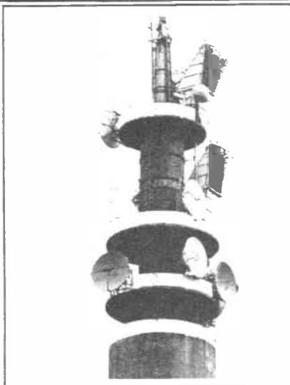
Above: it looms large and is imposing, the Stokenchurch antenna tower. But it's only a repeater for the London Post Office Tower, handling microwave trunk calls to and from the west of the country.
