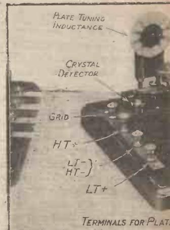
Fig. 4.—Crystal Detector Panel
