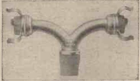
This is a most efficient device to which the ordinary headphones are clipped and the Gramaphix mounted on the tone arm of a gramophone. Straight or curved horns are supplied to fit from 6/6, the Gramaphix 10/6, making a complete loud speaker for 17/-.
