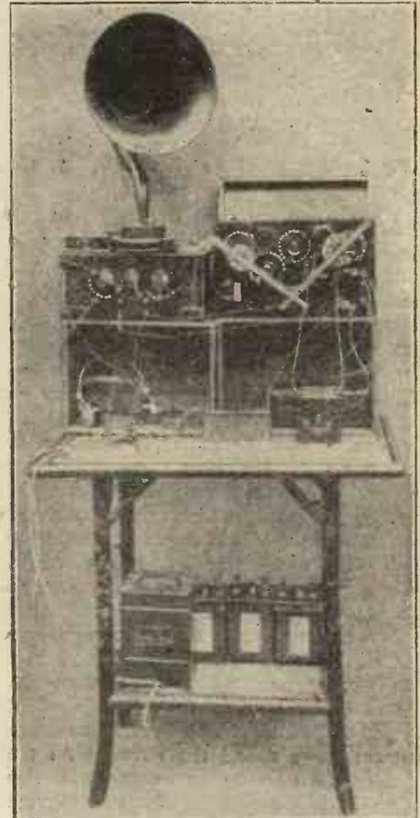
A Short-wave Receiver and Five-valve Amplifier made by Mr. H. G. Ede (Islington) from instructions in the "Work" Handbook "Wireless Telegraphy and Telephony."
