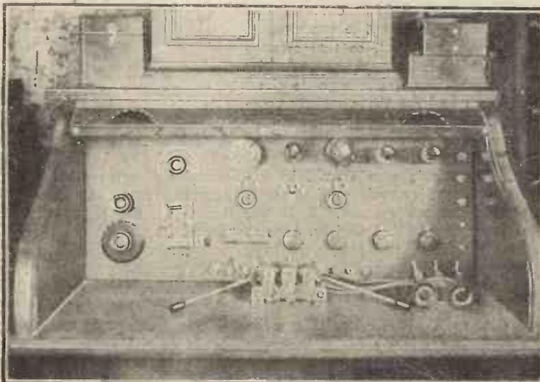
How a receiving set can be conveniently mounted in a roll-top desk is shown in the above photographs, which depict a station built by Mr. F. Worrall, of Bolton. The illustration on the left shows the whole receiving station and that on the
