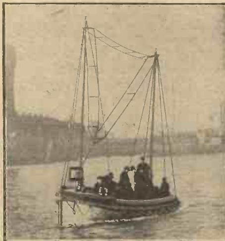
Marconi Installation on a Ship's Lifeboat.
