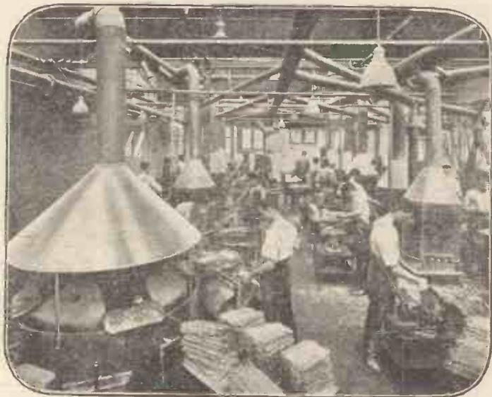
The Grids are cast in pairs by hand-operated machines.
