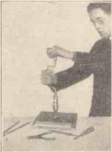
Much time and labour can be saved in cutting large holes in ebonite panels for meters, valve windows, etc., by the use of a disc cutter held in a brace.
