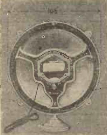
The two Squire loud-speaker cradles and cones illustrated here are a definite improvement on the average type of loud-speaker hitherto available for receivers. The Squire polished aluminium cradle is very light, does not cause aerial interference, and is notable for its rigidity and compactness.
