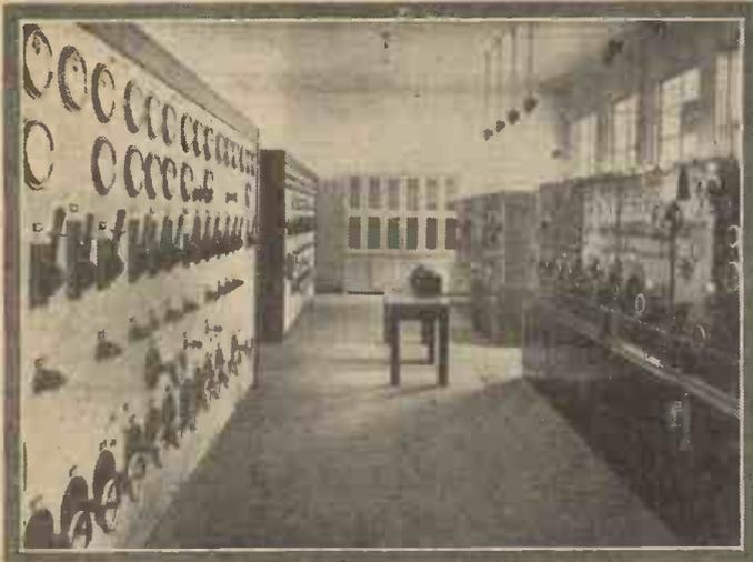
The transmitting apparatus and switchboard of No. 2 Short-wave Station
