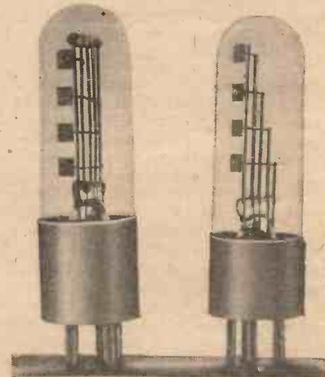
Multiple-target neon lamps used in the Jenkins receiver
