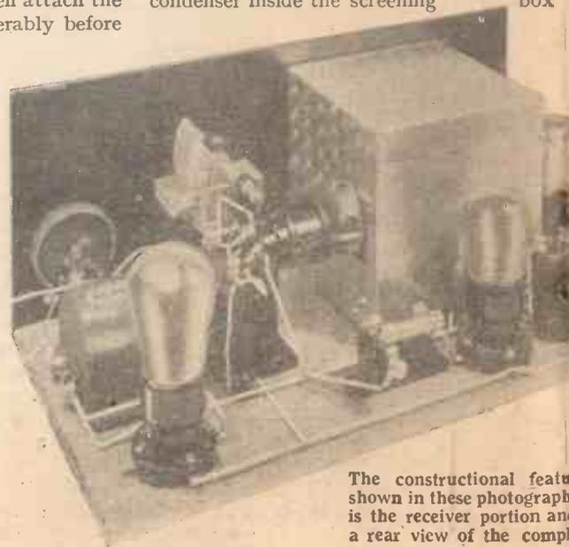
The constructional features shown in these photographs are the receiver portion and a rear view of the complete set.
