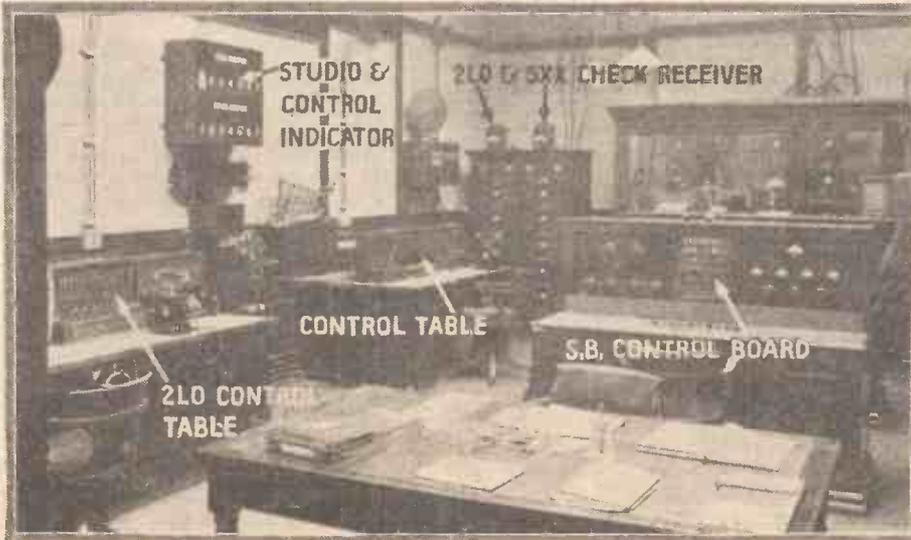
This view of the inside of a control room clearly explains the various units
