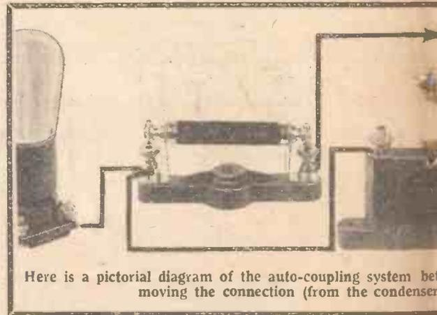
Here is a pictorial diagram of the auto-coupling system before moving the connection (from the condenser)
