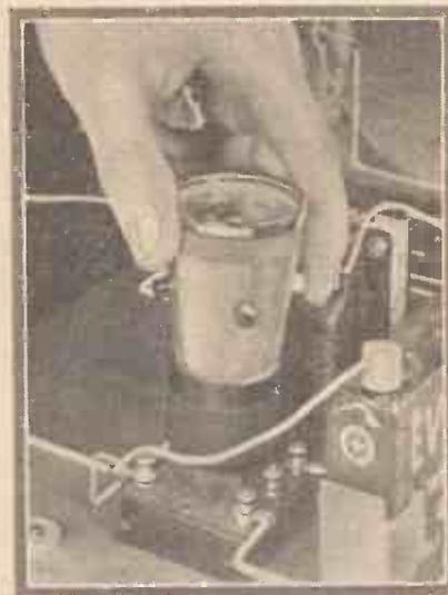
The C.F. Radio Controller which plugged in to a valve holder shows any faults in the H.T., L.T. or grid circuits
