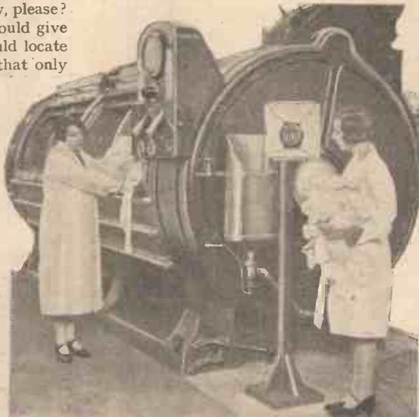
Calling to the washing! This giant washing machine at the International Laundry Exhibition in London is started and stopped by means of amplifiers and a microphone. The “mike” is in the foreground
