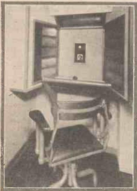
In the lower part of the opening one sees an image of the person at the distant end. From a point just above it, the scanning beam is directed to the face of the speaker, and the reflected light is picked up by photo-electric cells visible through the glass plates at sides and top
