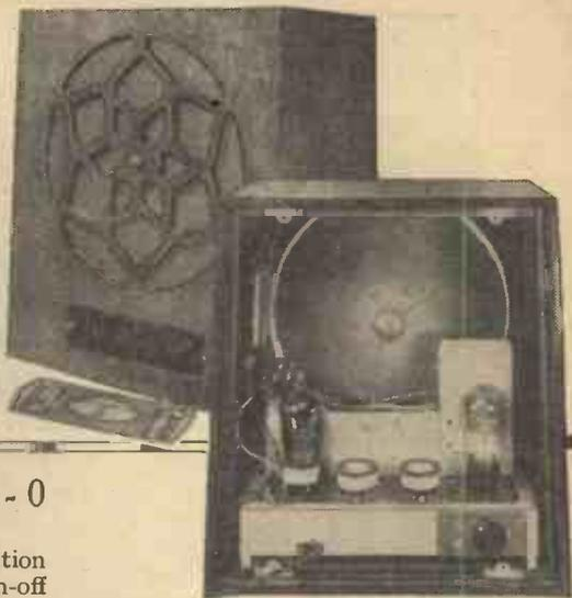
ENTIRELY novel in design is the latest product of the Columbia Graphophone Company, Limited. This is an all-electric two-valver for A.C. mains. It can be used on all supply voltages between 100 and 250 volts, provided that the right model is ordered. Still another model is available for D.C. mains supplies.
