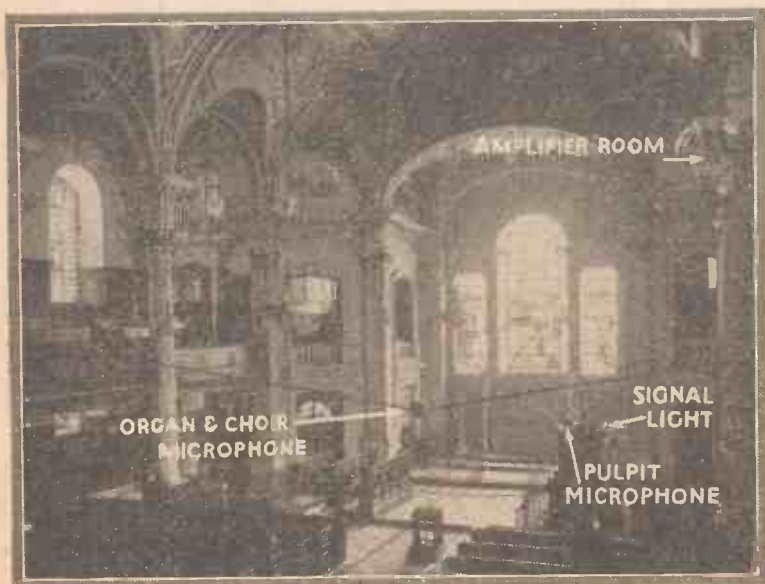
This view of the inside of the famous London church, from which broadcasts are so frequently made, shows where the two "mikes" and the signal light are placed
