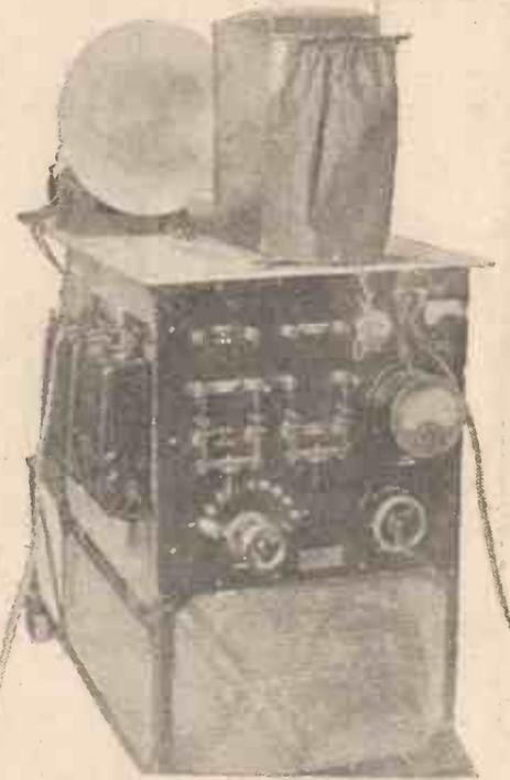
This is the standard type of transmitter which has been used until recently
