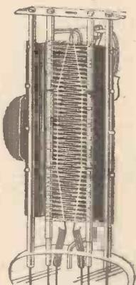
Showing the ultra-rigid assembly, interlocking mica bridge and very large electrode area of HL2.
