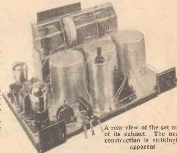
A rear view of the set out of its cabinet. The neat construction is strikingly apparent
