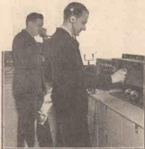
Inside the "O.B." van. Duplicate amplifiers are carried in the travelling van which the B.B.C. uses for outside broadcasts, and an engineer is here checking up the tone quality on one of the lines linking up the van with the control room
