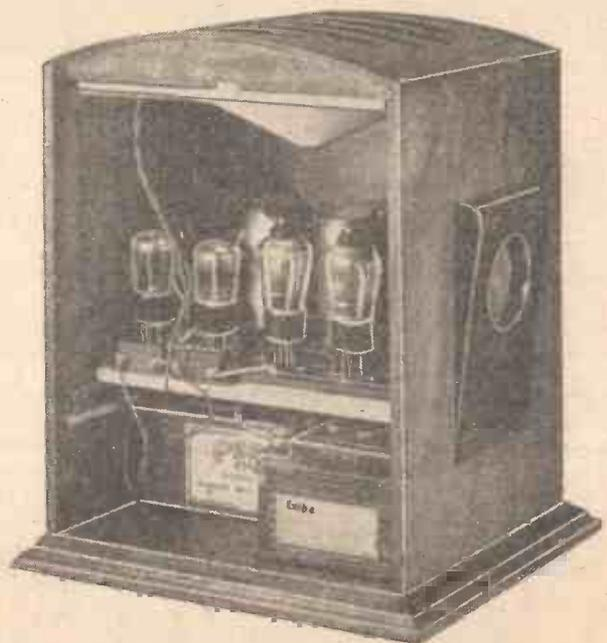
Note the ample space available for the batteries
