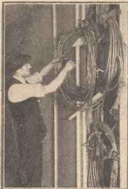
The hundreds of cables linking Broadcasting House's studios with the control room are carried in this conduit
