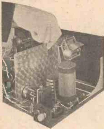
Do not adjust the set so that the selectivity factor is greater than is really necessary for reception conditions at the time. By slacking off the pre-set condenser, for example, one can in many sets make the tuning unnecessarily sharp and this may affect the quality on the high-frequency side
