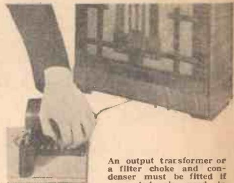
An output transformer or a filter choke and condenser must be fitted if a pentode is used in your set, and is an advantage even when an ordinary power valve is used. Here a choke and condenser are being connected up between the set and the speaker
