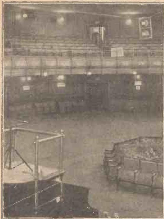
Here is another form of microphone suspension in the Queen's Hall. The twin "mikes" can be seen at the top right, together with the suspension cables and the microphone lines
