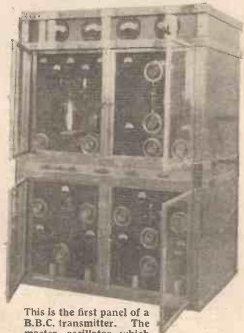
This is the first panel of a B.B.C. transmitter. The master oscillator which keeps the wavelength constant is in one of the right-hand compartments
