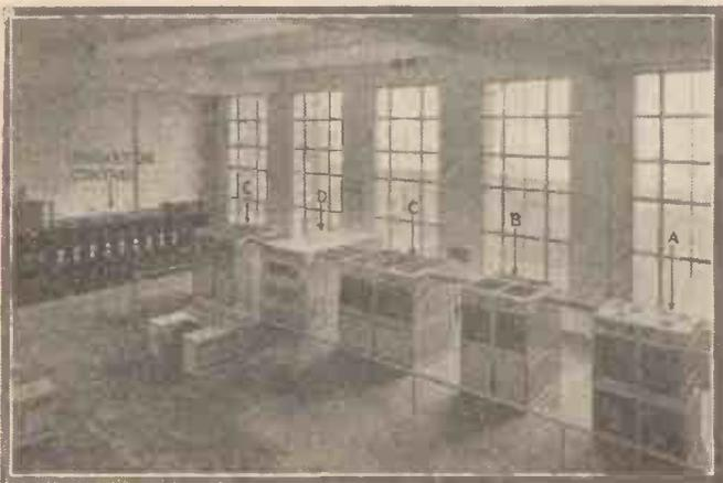
Here are the five panels of the North Regional transmitter. There are two C panels, these carrying the final water-cooled valves. The tuning coils are in the D panel
