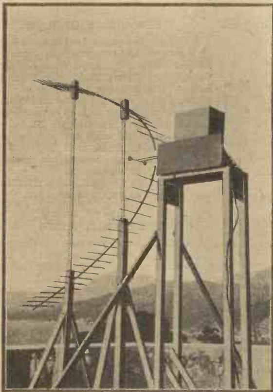
This is the special beam aerial used by Marconi in his recent experiments in Italy in sending signals on a wavelength of half a metre over a distance of twenty-five miles. This is the aerial at the receiving end
