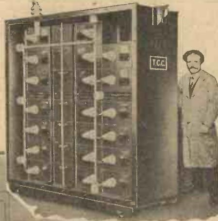
Some of the big condensers, rated to work up to 25,000 volts D.C., can be seen at the left, while (above) one of the operators of the station is holding one of the cases containing condenser banks.
