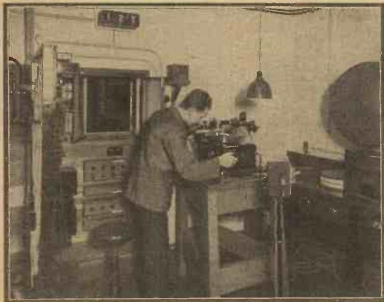
Behind the scenes at one of the recording rooms of the new H.M.V. studio centre in London. A wax is being made and the engineer is listening, by means of a speaker, to what is going on in the studio, which can be seen through the observation window in the centre
