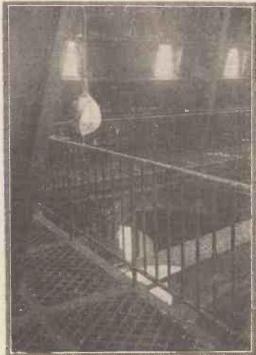
Broadcasting "Big Ben." Close up view of the suspended microphone in the gallery above the bells of "Big Ben." The instrument is enclosed in a protective cover of rubber
