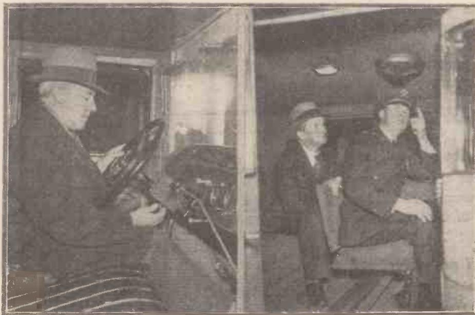
(Left) The receiver used in new police cars in New York is remote controlled, from the small box clamped to the steering column. (Right) Each car is fitted with a speaker in the roof and this puts the "speed cops" in direct touch with police Headquarters, where the movements of criminals are reported by telegraph
