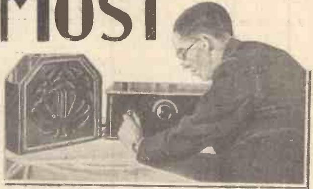
**I**N all but the biggest of sets reaction is still employed. Its main function in, say, a three-valver is to add to the high-frequency amplification obtained from the valves. A well-designed reaction system, by which I mean one that will enable the point of oscillation to be approached smoothly and without erratic "plops," is often almost as good as another stage of high-frequency amplification.
