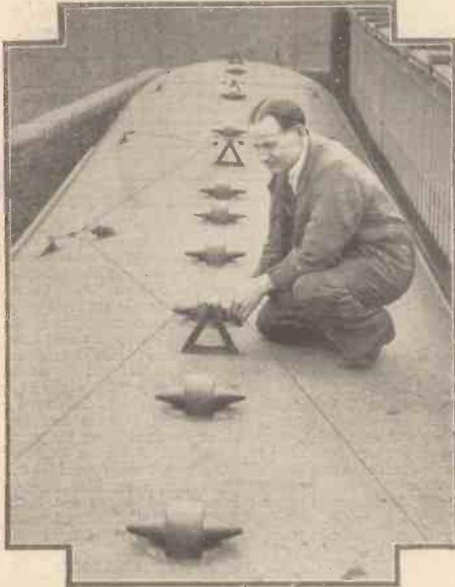
Owing to the popularity of radio on trains, the L.N.E.R. have now fitted two of the Scottish expresses, working on the East Coast route, with radio gear. This photograph shows the double aerial equipment on the roof of one of the trains
