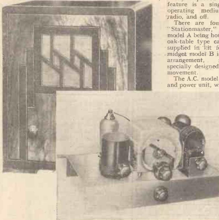
One of the new "Radio for the Million" receivers, and (inset) the chassis, showing the neat construction. Kits of parts are supplied for these sets
