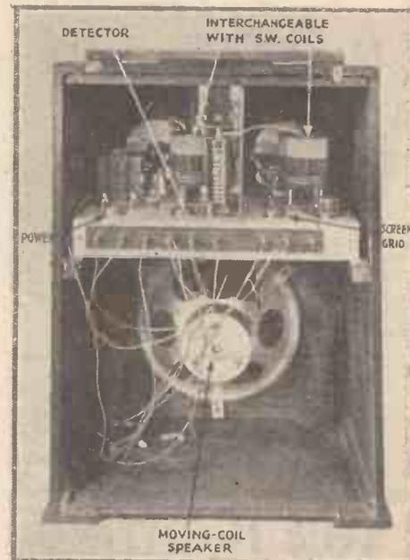
The Meteor Three is metal-chassis built and most of the wiring is underneath the base
