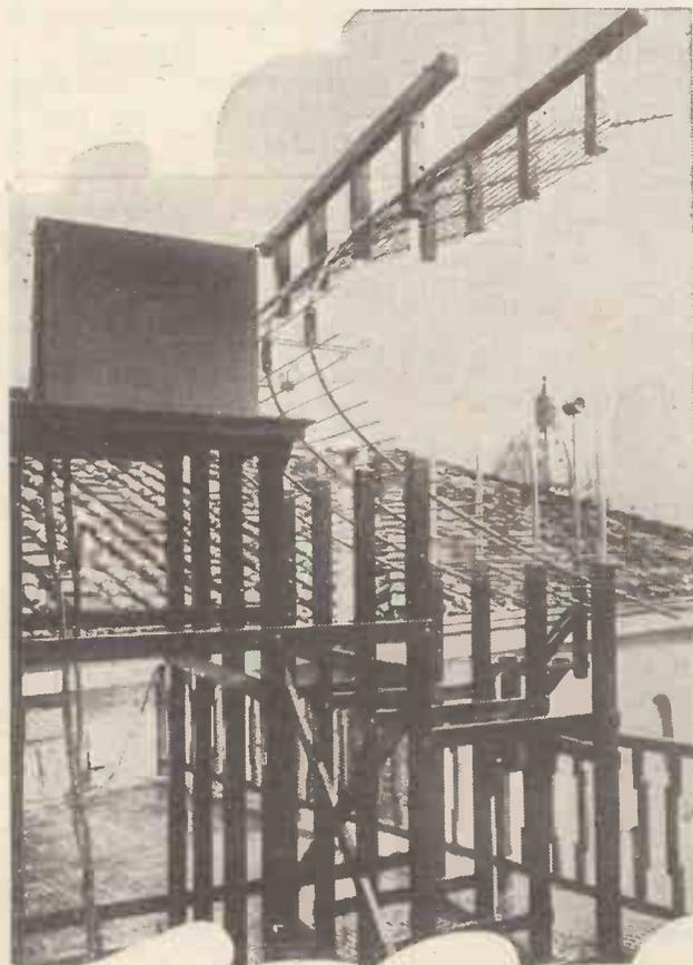
Micro-ray radio for the Pope! This is the beam aerial reflector in the Vatican of the special ultra-short-wave transmitter which is used for communication with the Pope's Palace, eighteen miles away.
