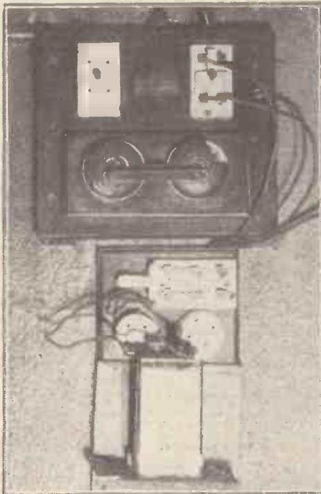
Fig. 4. Here the battery is shown connected near the meter so that all the current used in the house passes through it
