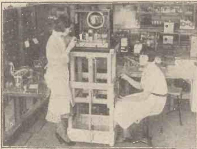
To meet the seasonal rush of orders, the H.M.V. factory has introduced many time-saving methods of production, including this lift arrangement whereby all parts of the set can be examined without undue fatigue
