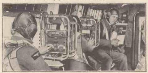
A Vickers-Victoria aeroplane equipped for wireless instruction, which is undertaken in the air. Five pupils use five separate receivers
