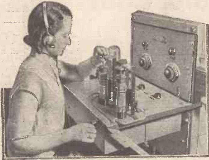
Matching coils is now a highly developed technique. Typical tests in the new Cossor works
