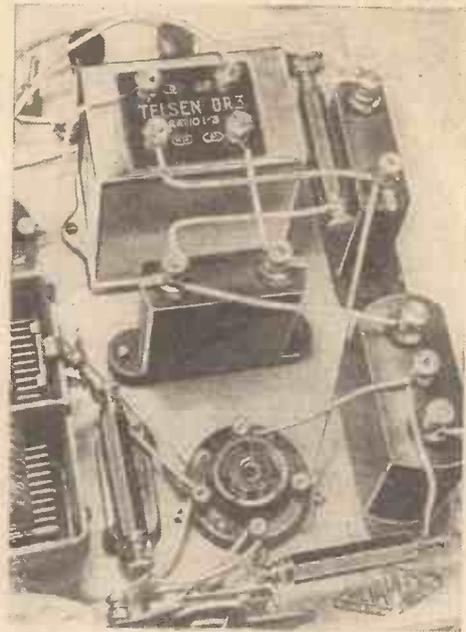
View of an important part of the set—the output stage of the 1934 Ether Searcher
