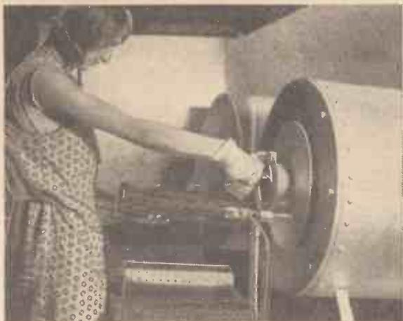
Electric furnace in the Cossor works for driving occluded gases out of valve electrodes
