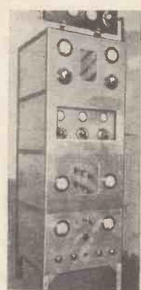
The 20-metre telephony station of W2GX, New Jersey; the power is 100 watts
