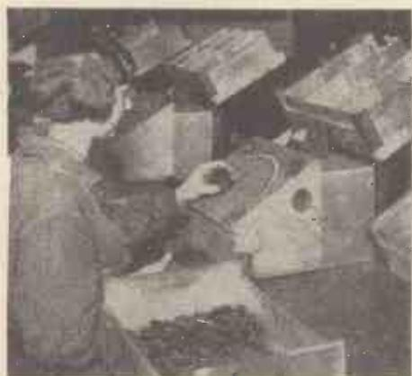
Testing the capacities of moulded fixed condensers
