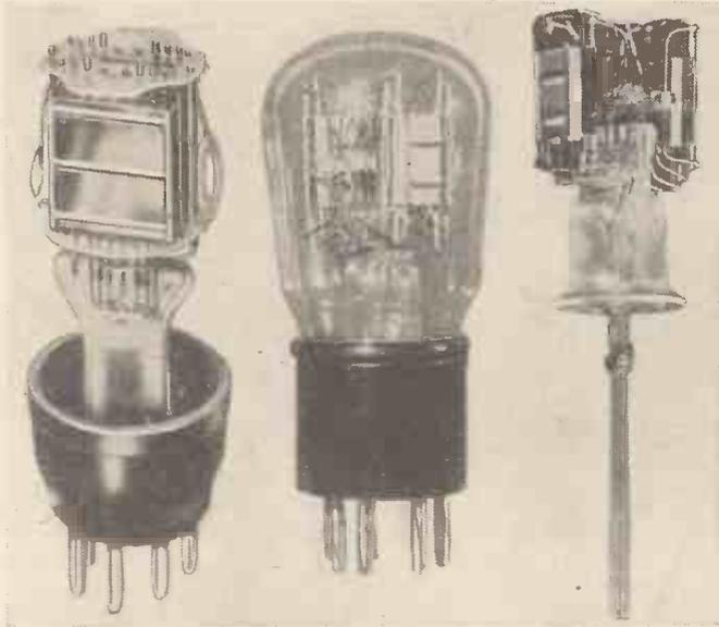
(Left).—Internal construction of the Marconi QP21 output valve. (Centre and right).—Two views of the 362 class-B battery valve
