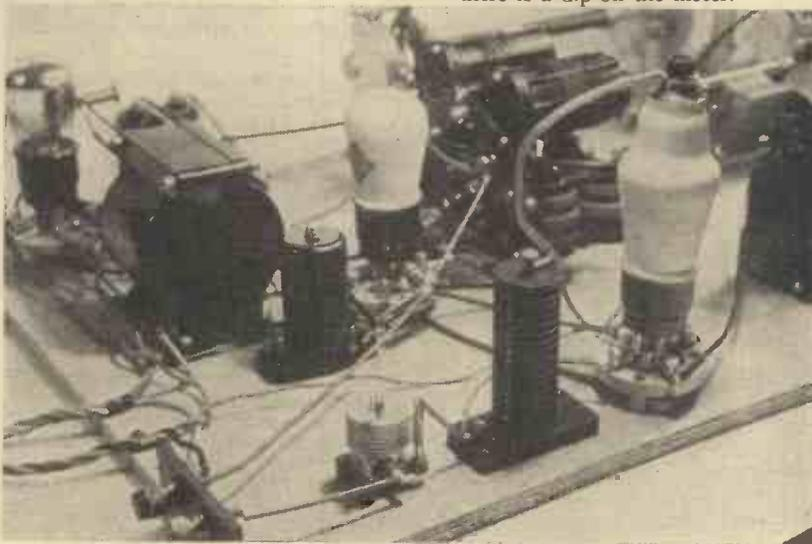
Another view of the Experimenter's Short-waver, a hook-up that employs an all-wave tuning coil and many special features
