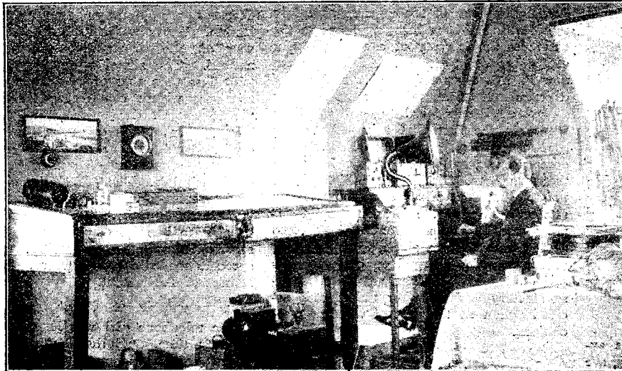
General View of the 5 LP Wireless Den.
