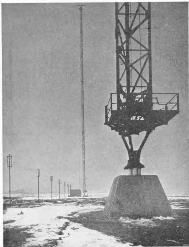
FEEDER LINES AND THE INSULATED BASE OF AN AERIAL MAST
