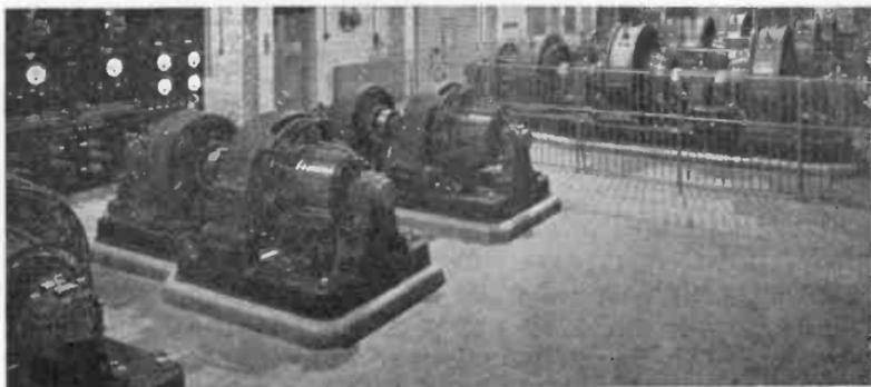
THE MACHINE ROOM—FILAMENT CURRENT GENERATORS (LEFT) AND
