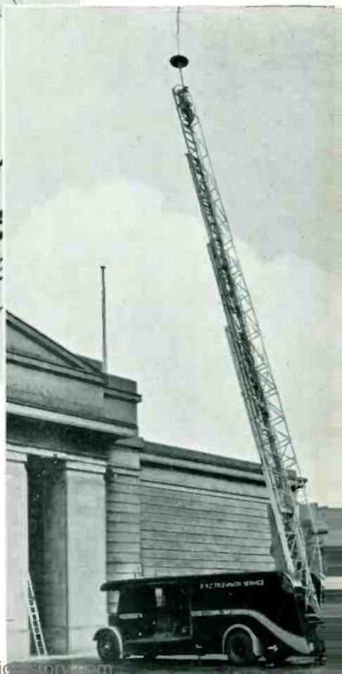
This combined aerial, transmitter and power vehicle is used for transmitting television pictures by radio from places where no cable link is available.
