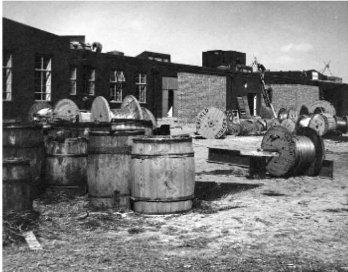
180 tons of equipment contained in nearly 600 cases ranging from 200 lb. to 3<sup>1</sup>/<sub>2</sub> tons were handled in the goods station at Woofferton railway junction. These had to be transported to the site and off-loaded before installation work could commence. *(Picture on left shows the scene outside OSE10 taken in 1943)*
