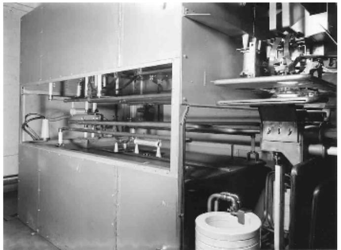
S81 was a total rebuild to a design by Mr. B. N. MacLarty which was never totally stable in operation. Instead of a push pull triode circuit with a neat Scott transformer filament supply it was single ended with a dummy valve. This meant that this one sender had a different final RF valve and required a large DC generator for its filament supplies. The standard RCA transmitters used two RCA 880 valves in the Final RF stage and two similar valves in the Modulator. In S81,
