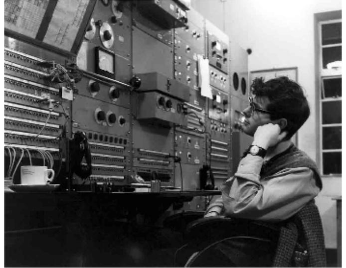
so that LFI could check at any time how his pet mechanism was behaving. This master clock drove all the other operational clocks displayed the building in a series circuit. Senders were switched off and on for the scheduled transmissions by the TAs who used the clocks in each sender hall.
