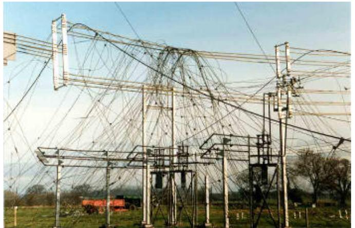
Doodle” spoiling their TV programmes. *(Sometimes arcing due to broken dipoles could cause TVI problems if not found. However this storm damage to A953 just before the March schedule change in 1987 was very obvious)*
