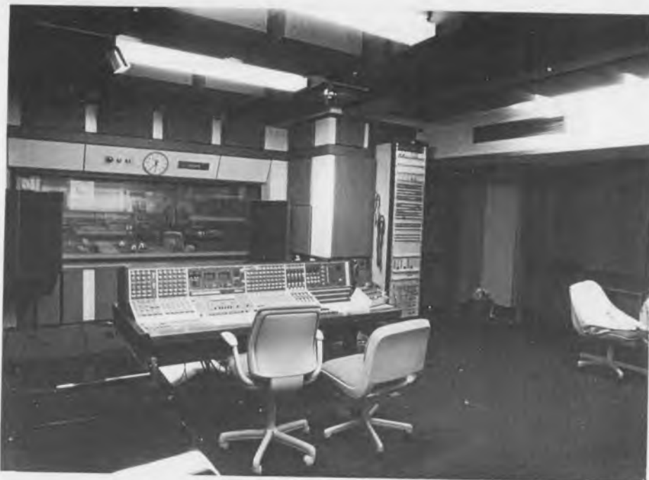
Control room of GP Studio, S7. One of the building's supporting pillars is cleverly concealed behind the jackfield to the right of the mixer desk
