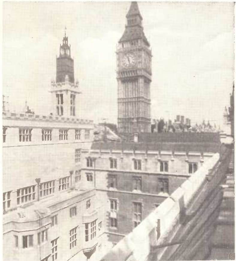
Clipsham stone was chosen for the rebuilding of the House of Commons: apart from its colour and texture, it stands up well to the London atmosphere
