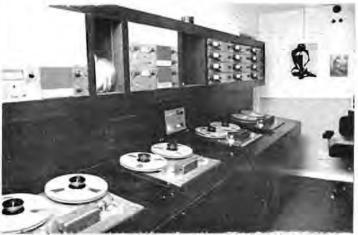
Trident's new Ampex 8-track tape machine, installed in a special tape machine room.
