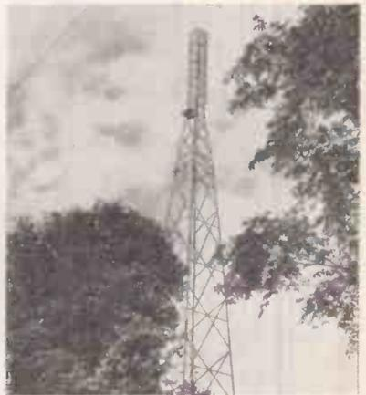
The Marconi mast and aerial, erection of which is completed, at the Croydon I.T.A. TV transmitting site. The aerial is a twin 4-stack Bnd III vertically polarised array. Meanwhile installation of the sound transmitter is complete, and the installation of the vision transmitter is going according to schedule.
