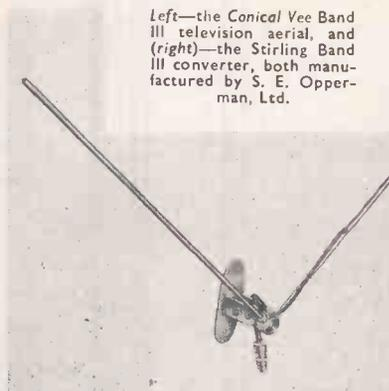
Left—the Conical Vee Band III television aerial, and (right)—the Stirling Band III converter, both manufactured by S. E. Opperman, Ltd.
