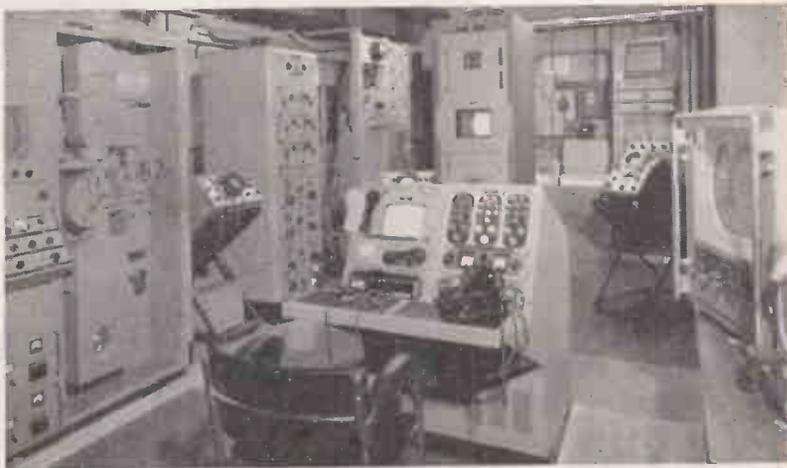
A view of the B.B.C. experimental colour television studio at Alexandra Palace. In the centre is the control console with three-tube colour picture monitor. On extreme right is a radio check colour receiver.
