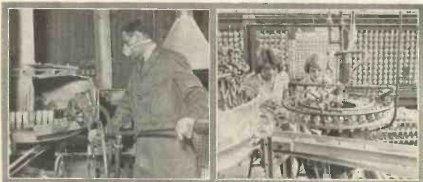
Two processes in the making of valves at Ediswan's Brimsdown factory. Left is the metal spraying equipment and, right, capping machines.
