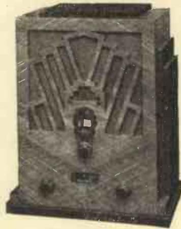
Double band pass tuning is employed in this three-valve British General set which can be examined on Stand No. 12a.
