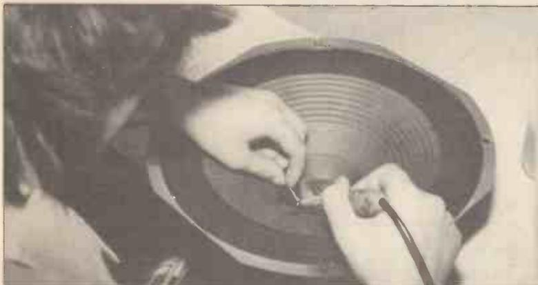
Soldering wire connections to cone.
