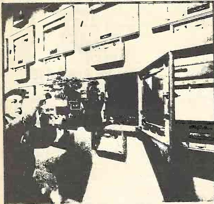
Fig. 1. Chart recorders are used in many varied applications. The panels of this control room contain a number that are used by the operators to see how the process is behaving.
