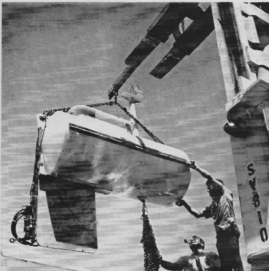
The forerunner of a buoy system which would maintain a continuous watch on water pollution levels is being tested in San Francisco Bay by Lockheed Missiles & Space Co.
