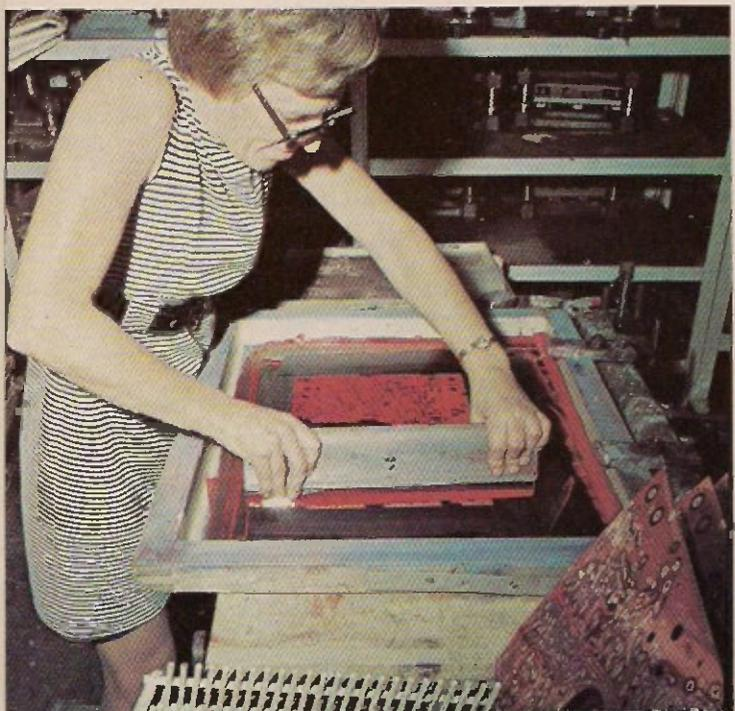
Silk screen process imprints circuit pattern onto board prior to etching.
