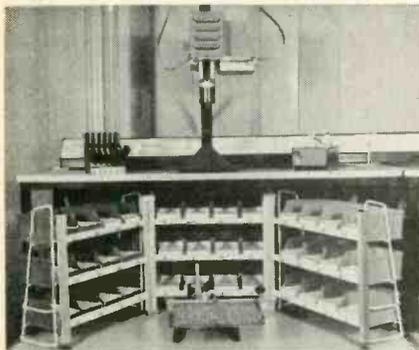
The system, developed over a number of years, is capable of indicating 100 component locations and can use three different display systems. The small and local beam of projected light for each compartment is comparatively bright, so that the operator can work in low ambient lighting. This reduces fatigue and so leads to greater efficiency. Complete boards can be economically manufactured in one operation, eliminating the costs associated with breaking down the assembly into simple stages.
